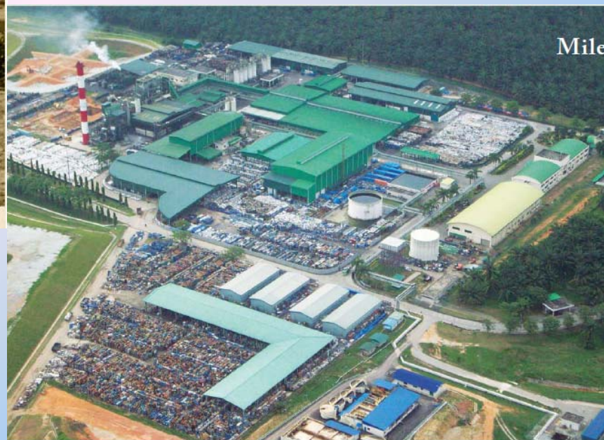
Aerial view of the Integrated Toxic and Hazardous Wastes Facility at Bukit Nenas, Port Dickson, Negeri Sembilan
